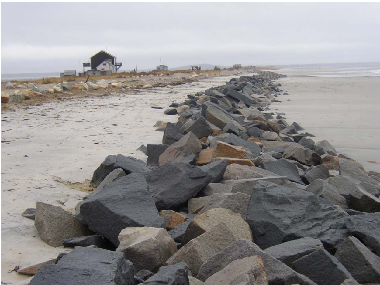
Photograph 1: Existing stone dike (view to the north).
