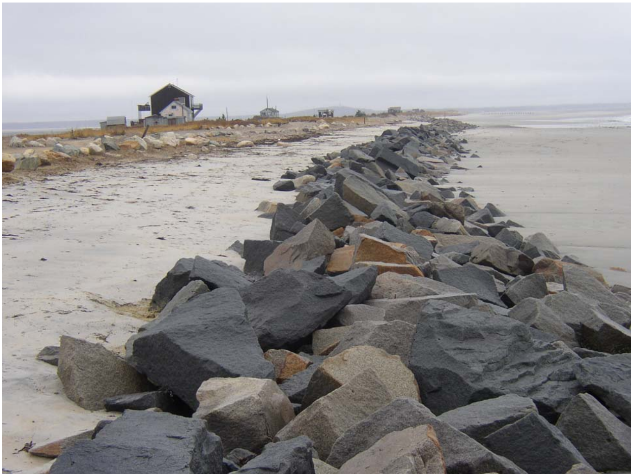
Photograph 1: Existing stone dike (view to the north).
